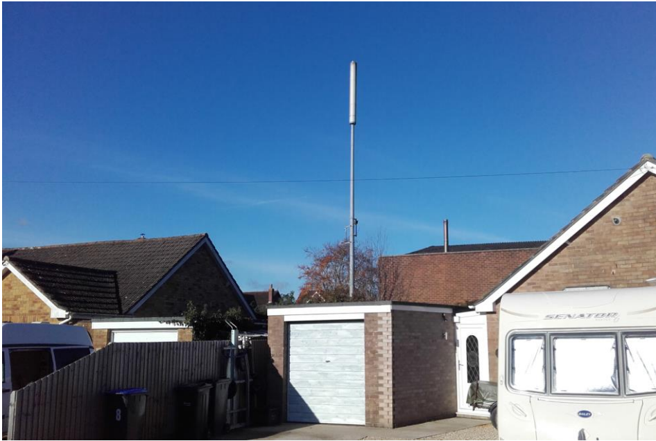
Existing Mast to rear of Springfield Crescent (to be removed)
